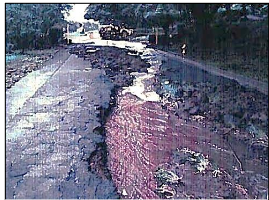
Damages to Kili Drive after January 2011 storm
