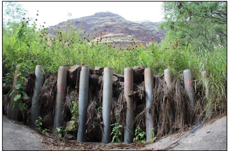
Three-foot debris poles filled with rocks to the top
