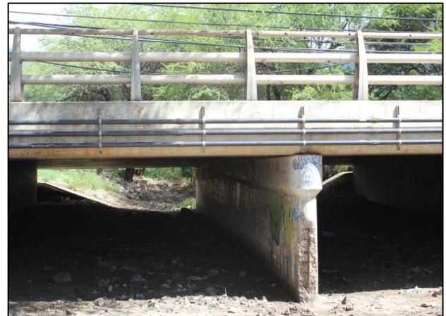
Existing Eku Stream Bridge
