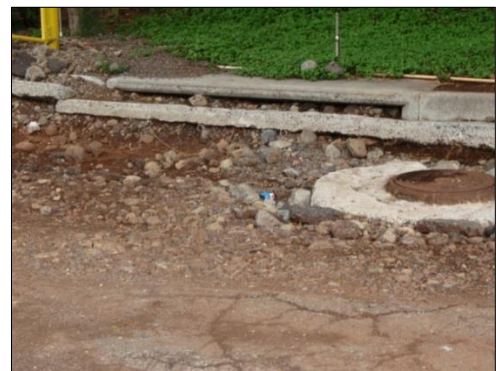
Storm drains clogged with rocks
