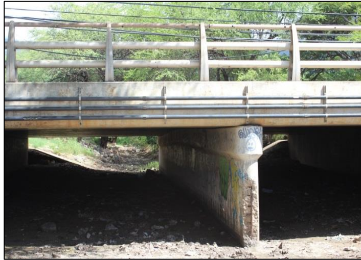
Eku Stream Bridge along Farrington Highway
