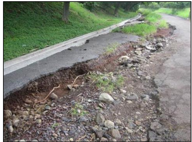
Road damage on the BWS Reservoir Road due to flooding
