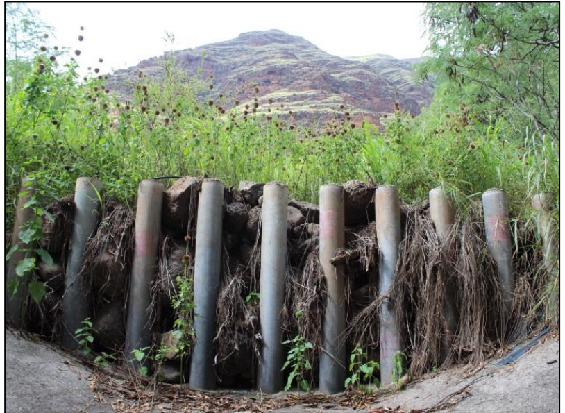
Three-foot debris poles filled with rocks to the top
