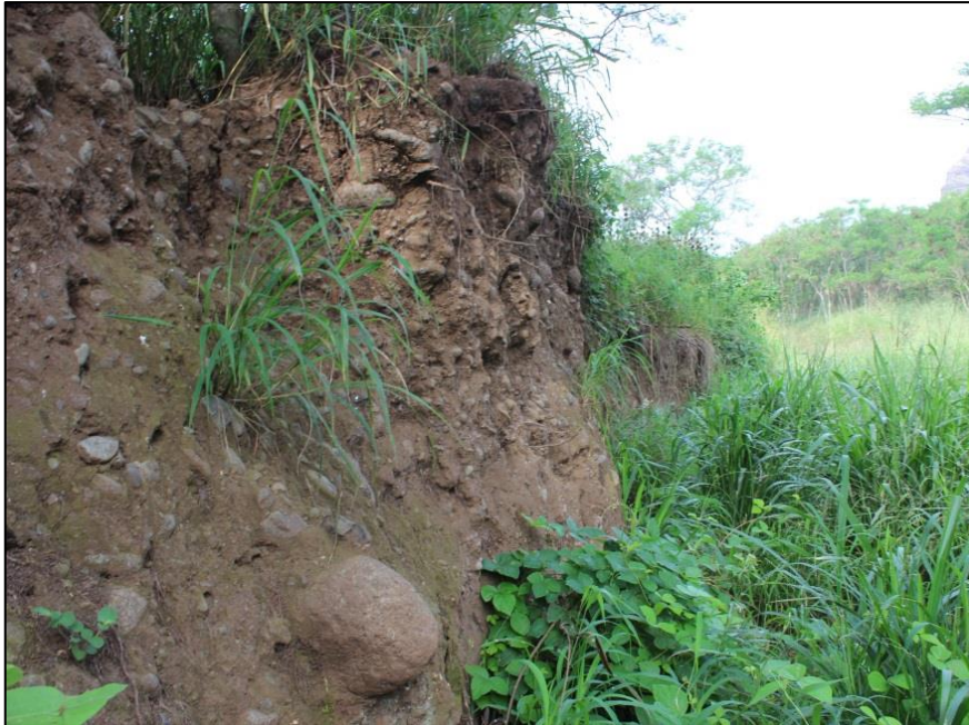
Signs of erosion and scour on the existing earthen berm
