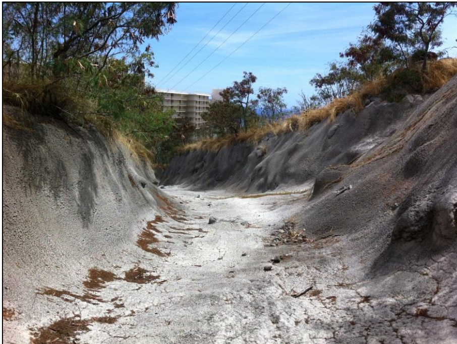
Existing channel behind Mākaha Valley Towers
