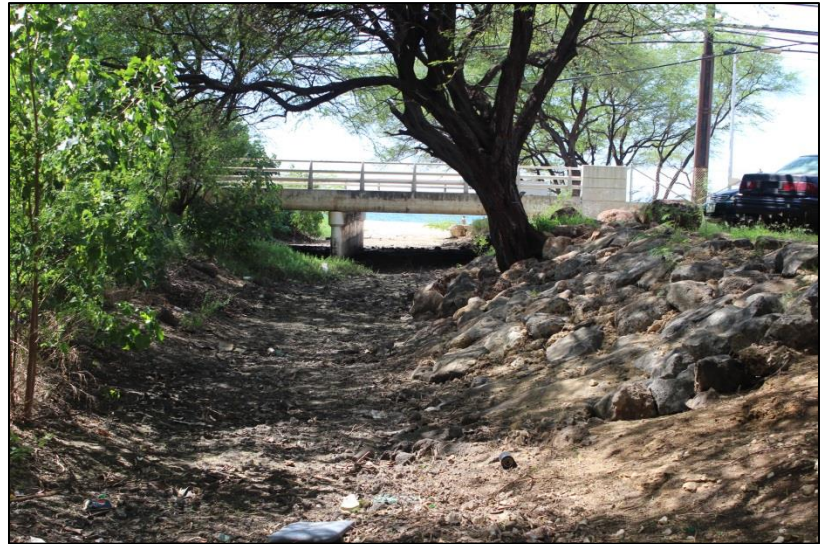
Eku Stream Channel near Farrington Highway facing makai
