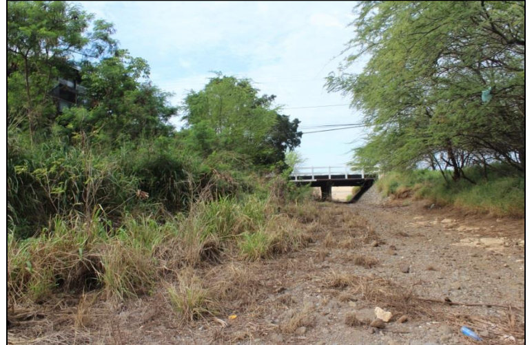
Existing Mākaha Stream Channel near Farrington Highway (facing makai)
