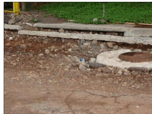
Storm drains clogged with rocks
