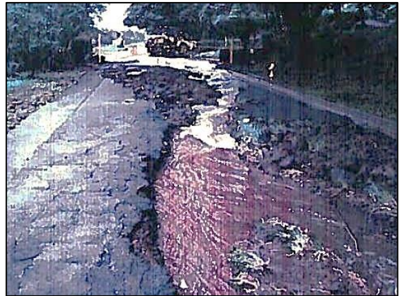
Damages to Kili Drive after January 2011 storm
