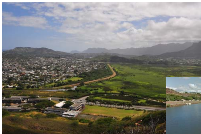
Kawainui Marsh Levee, Oahu
