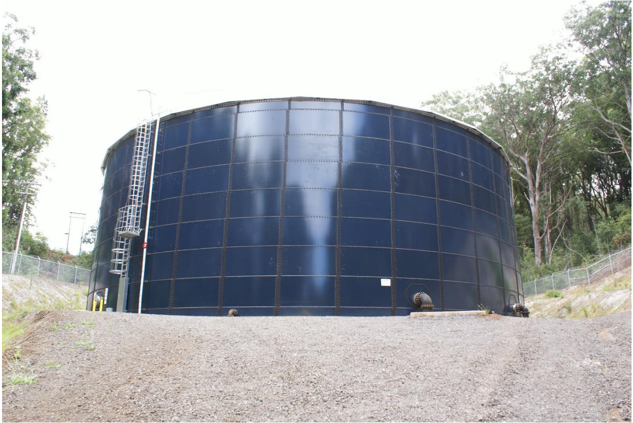
Modular glass lined steel tank on Lanai.
