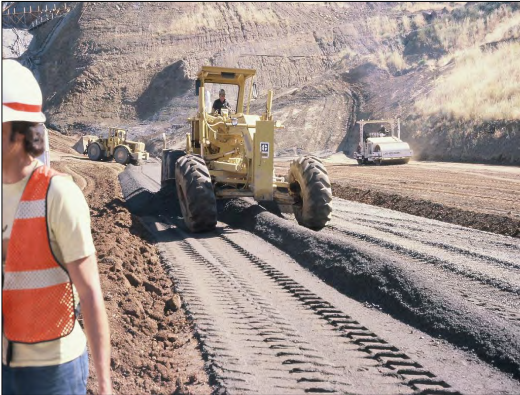
Figure 7-13. Spreading sand filter material.
