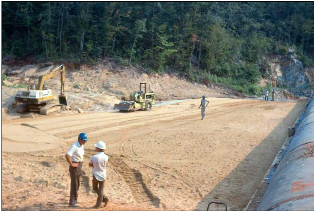
Figure 2-9. Fine filter being placed on the bedrock surface under the downstream shell of an embankment. View is toward downstream toe. Conduit is on the right of photograph. Exposed bedrock not yet covered is in background behind excavator. (Photo courtesy of NRCS, Alabama.)
