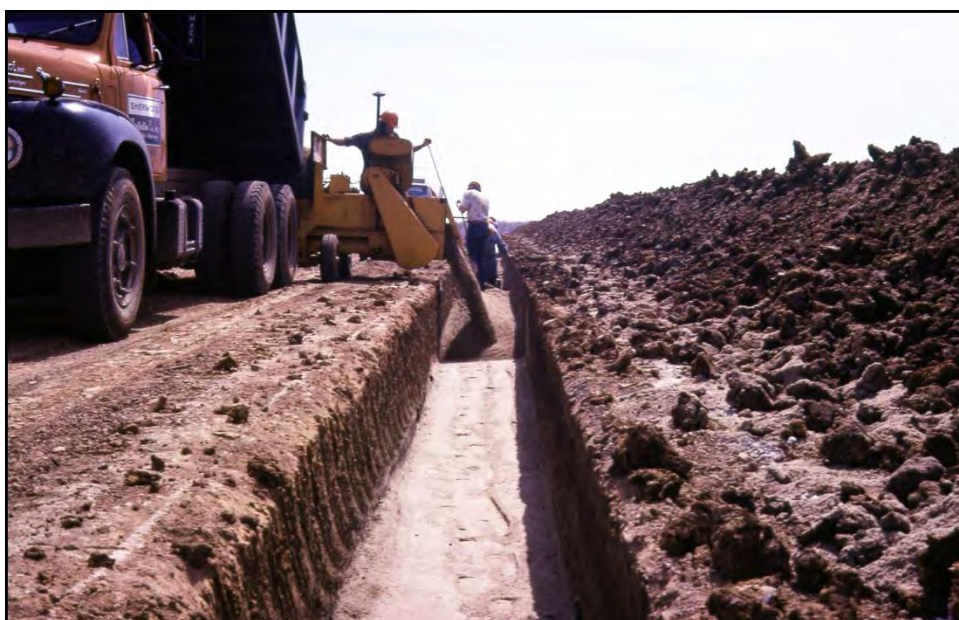
Figure 7-6. Trenching method – backfilling trench.
