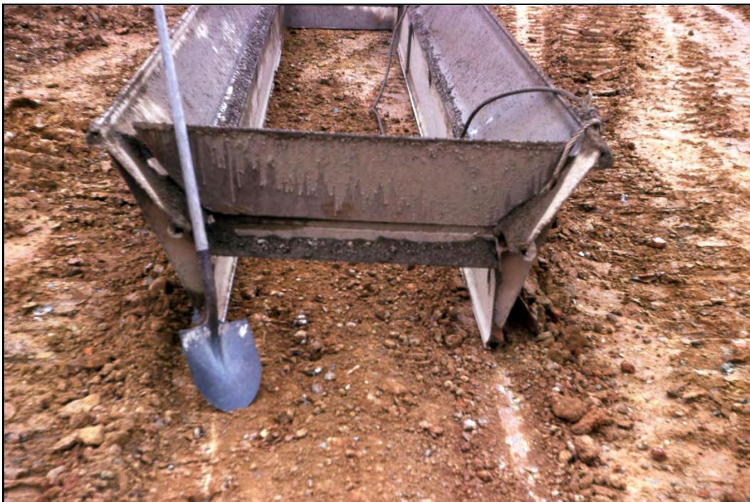
Figure 7-14. Basic single-bin spreader box.
