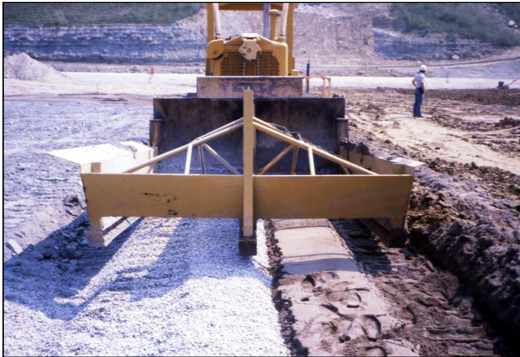
Figure 7-19. Double-bin spreader box fitted to dozer - front view.
