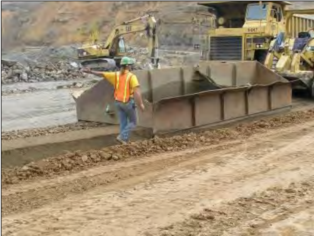
Figure 7-17. Towing spreader box.
