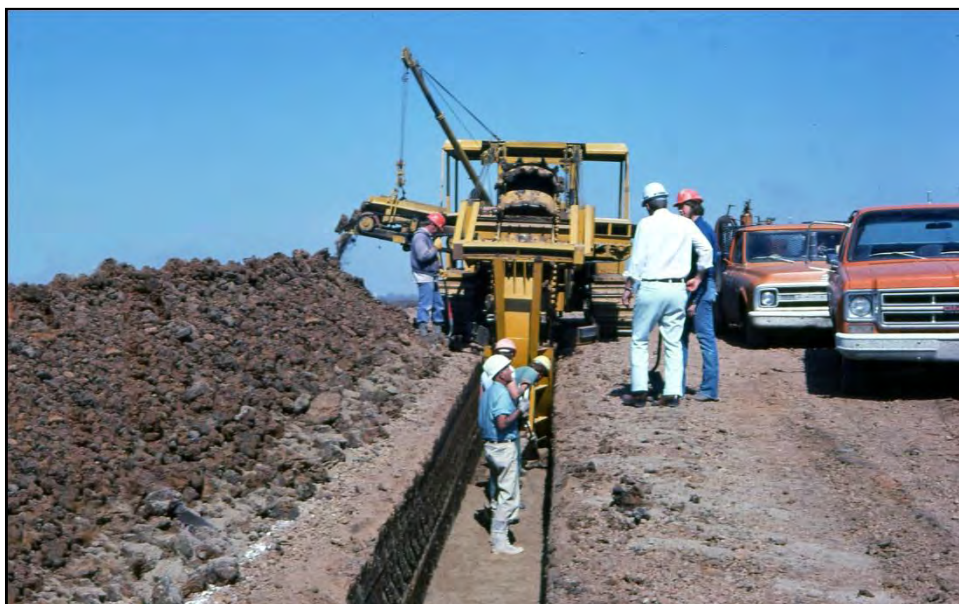
Figure 7-5. Trenching method – excavating trench.
