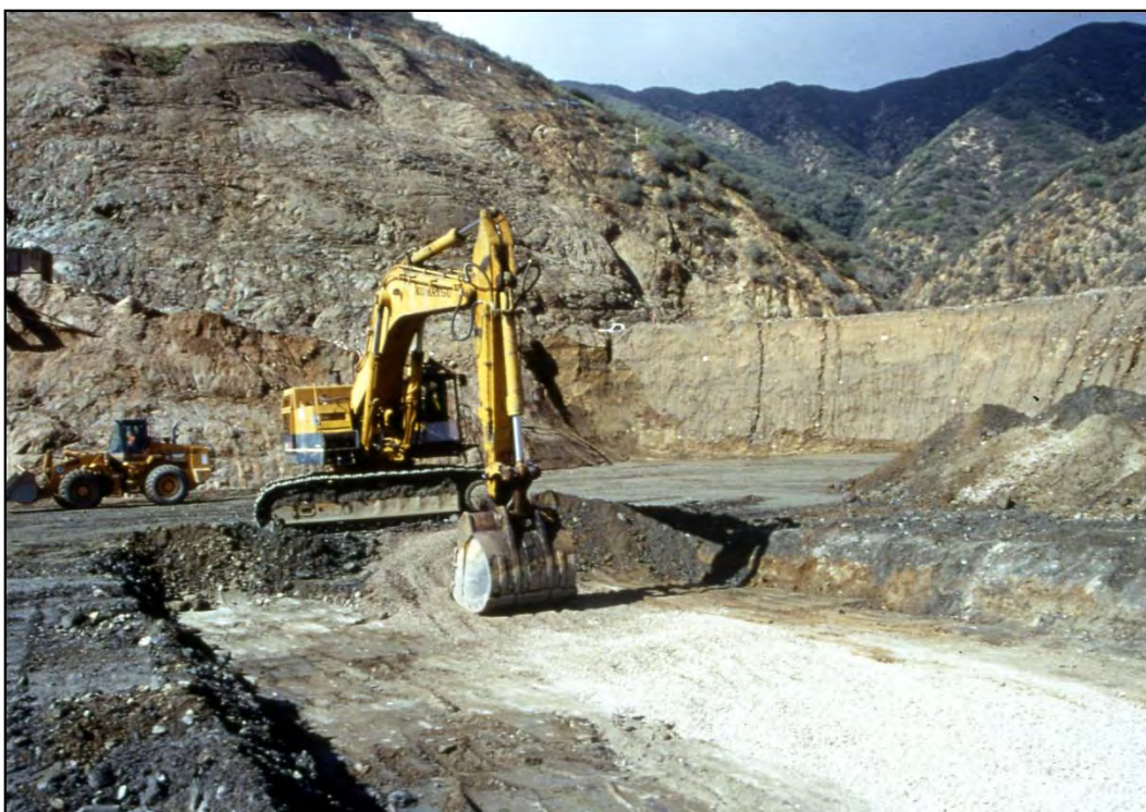
Figure 7-27. Excavation of filter material under equipment crossing.
