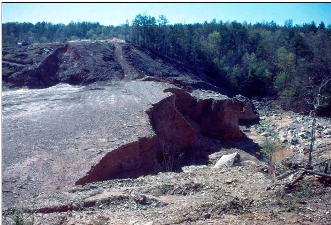
Figure E-2. View toward left abutment. This 50-ft-wide section of the dike overtopped and eroded a portion of the dike.
