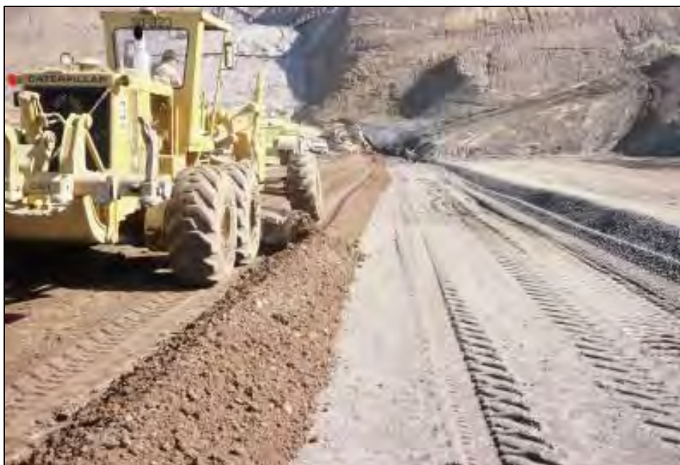
Figure 7-3. Windrowing impervious material adjacent to a filter/drain.
