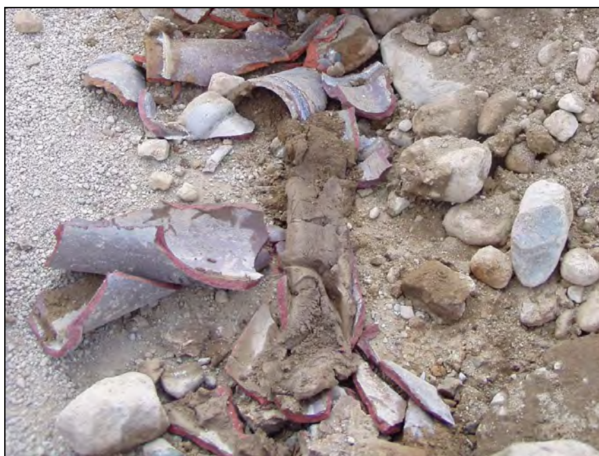
Figure 2-18. Clay tile pipe from 1916 as it was exposed during excavation. Note that the pipe was completely clogged with silt and sand.
