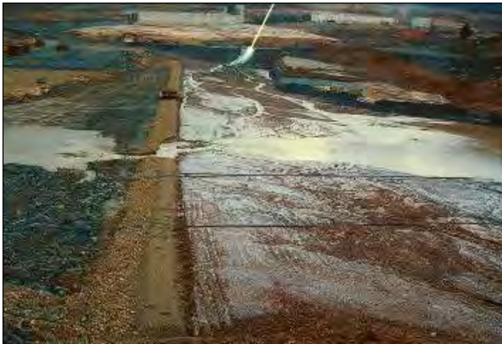
Figure 7-25. Surface water contamination of a chimney filter.
