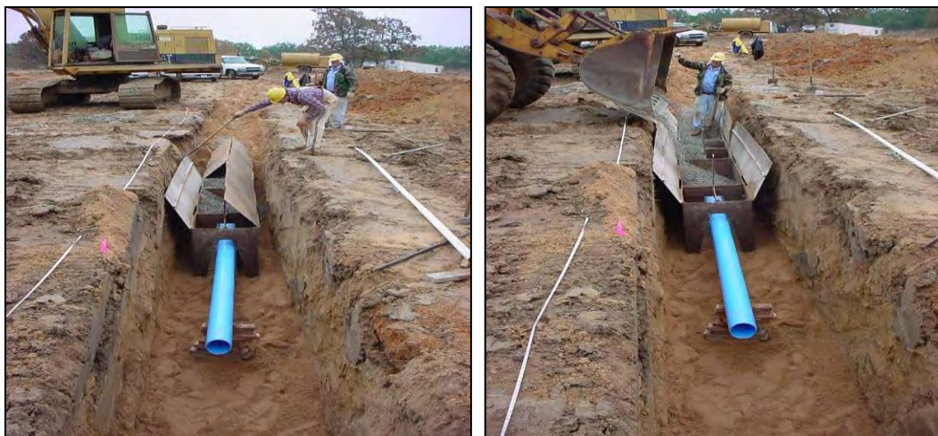
Figure 2-13. Rectangular cross section foundation trench drain with gravel filter surrounding perforated collector pipe and fine sand filter in primary part of drain. Boxes are contractor's ingenious idea of placing the coarse filter around the pipe. By closing the top of the box, fine drain fill can be placed and kept separated from the coarse drain zone.
