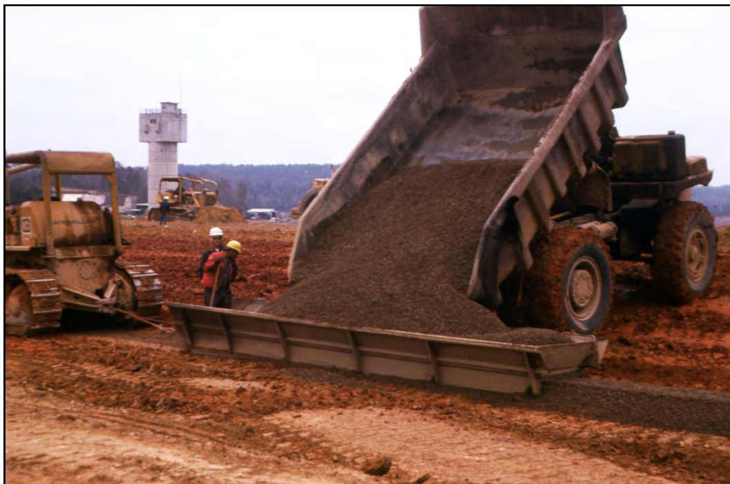
Figure 7-16. Dumping into spreader box.
