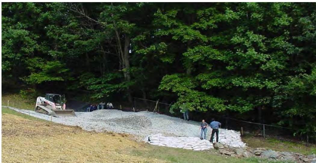
Figure L-26-2. Gravel drain being placed over seepage area.
