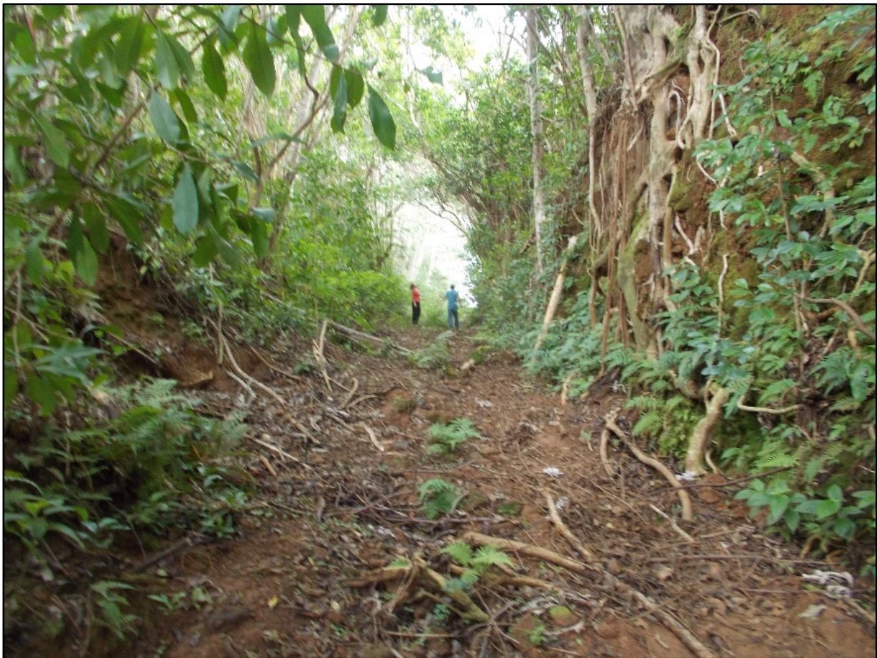
Figure 9. The narrow spillway channel as it approaches Kalihiwai Gulch. View facing east. Source: MASON, 2023.
