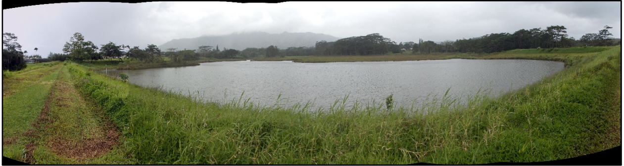
Figure 6: Kalihiwai Reservoir, overview facing south. This composite panorama shows the north section of the L-plan dam on the left, with the west section of the dam extending out to view to the right. Source: MASON, 2023.
