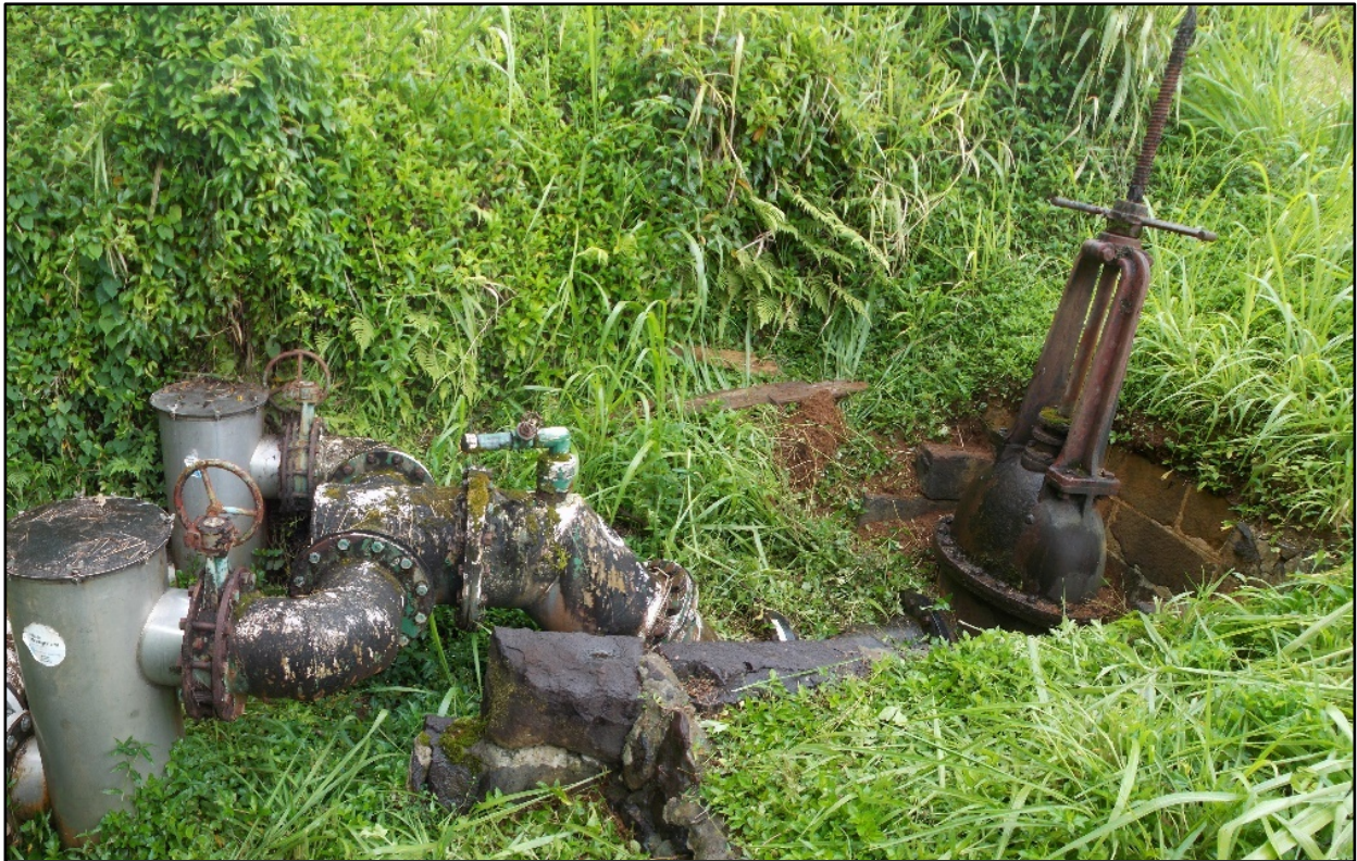
Figure 10. The historic outlet aperture is stabilized by coursed, quarry-faced lava rock masonry. Note the large metal gate valve at the right and the metal piping with two filters extending to the left from the gate valve. View facing southeast. Source: MASON, 2023.
