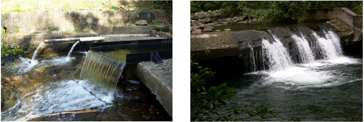
Figure 8: Over hanging diversions on Honopou Stream, Maui (left) and on the middle reach of Waihe'e Stream, Maui (right). Notice how the water free falls and leaves no pathway for upstream migration.
