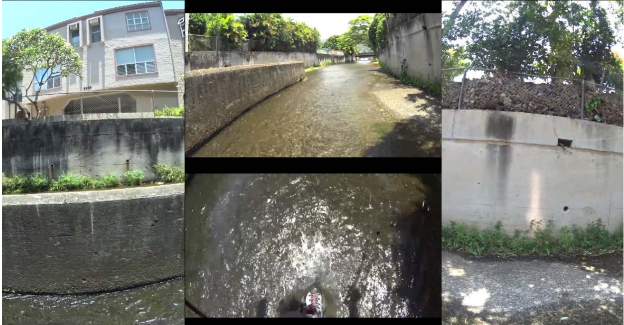
Figure 47: Channelized segment in Manoa Stream. Low-flow channel would begin just above wall in middle of stream.
