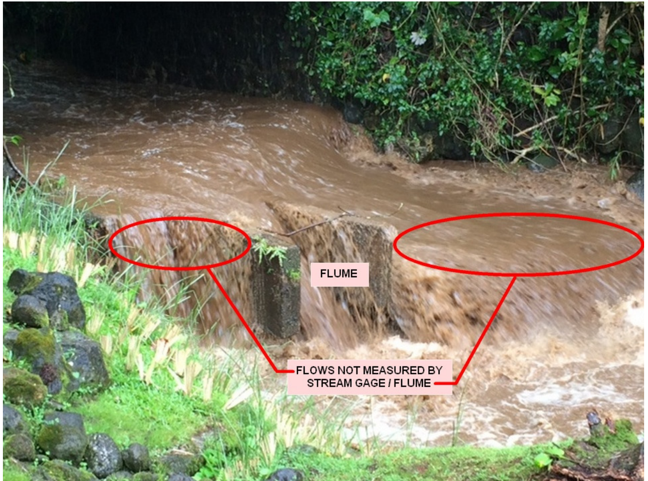
Figure 2 – Waiakeakua Stream Gage / Flume During Storm Conditions
