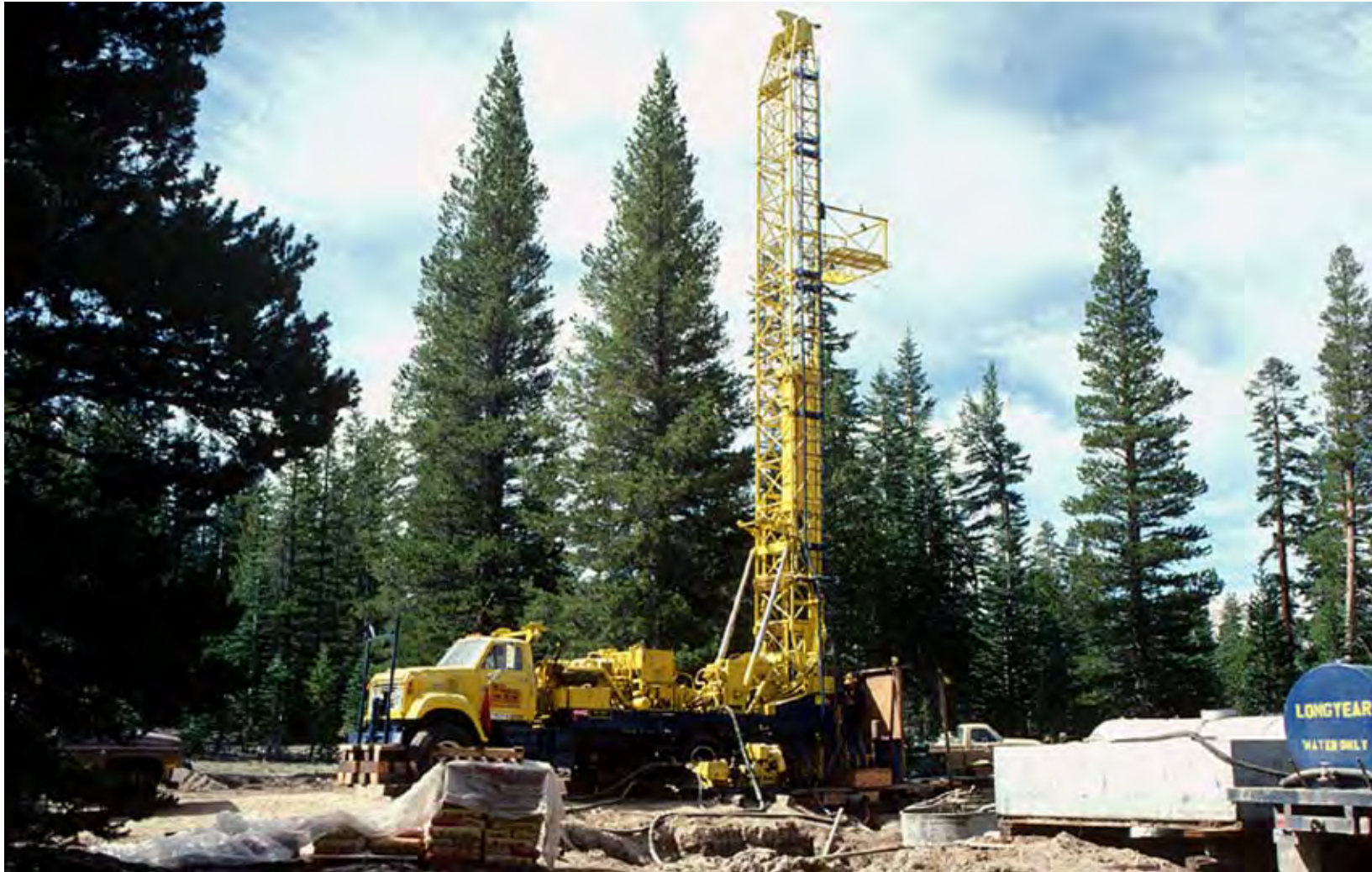
Figure 3.4: Drilling of a temperature gradient well.
